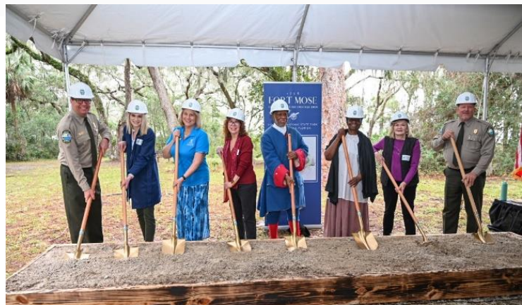
The groundbreaking for Fort Mose, Friday, January 19, 2024
